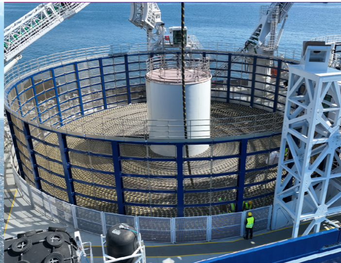
Offshore cable installation underway
