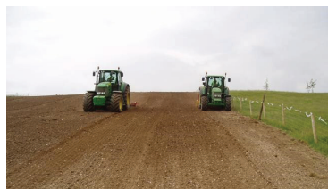
Land reinstatement after cable laying
